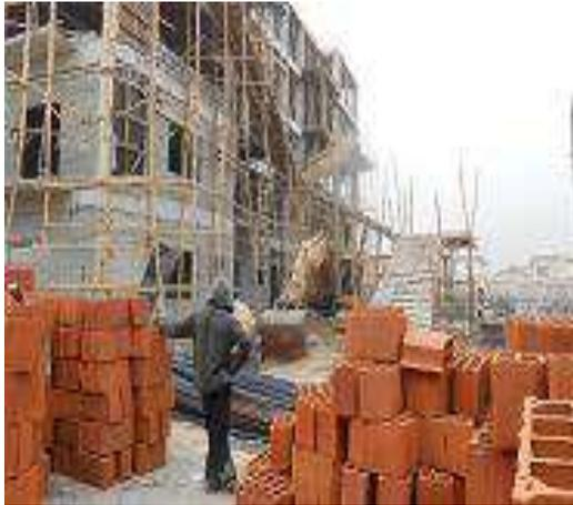
**Figure 4.2: Piling of material arbitrarily**
