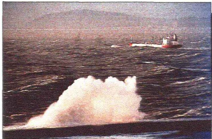
Waves pounding the breakwater wall, the spray reaching a height of about 20 meters.
