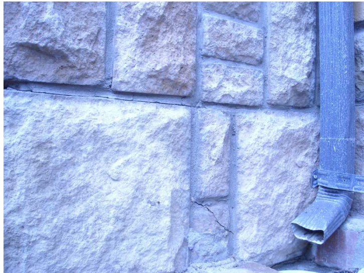
Figure 4-20 Poor storm water drain construction
