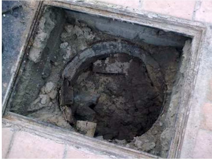
Figure 4-20 Poor storm water drain construction
