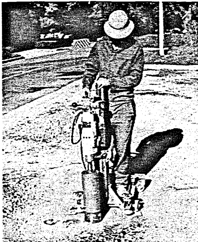
Figure 5-11: Coring in progress
