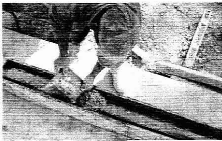
(a) placing of concrete in moulds
