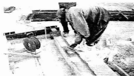
(c) finishing open ends of concrete
