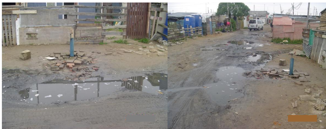
Figure 2-1: Greywater runoff at standpipe along the street
