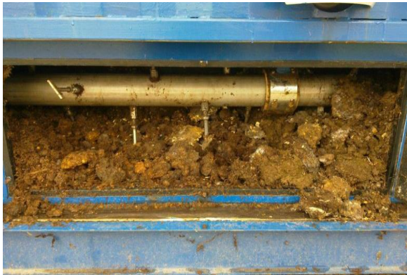
D3: Desiccated HF in the male toilet vault
