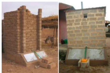
Figure 2.3: UDT Double vaults (Crepa, 2007)
