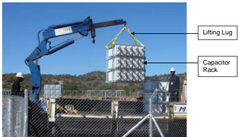
Figure 5.8: Crane removing capacitor rack from truck
