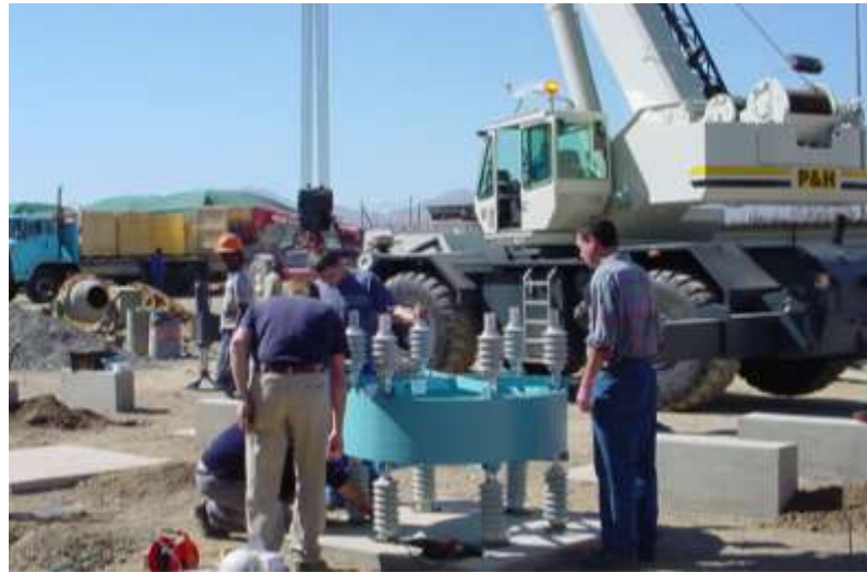
Figure 5.14: Reactors being assembled at site
