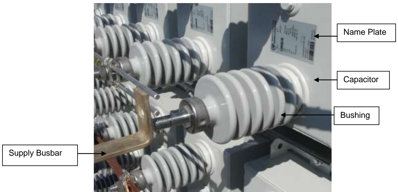
Figure 5.10: Connecting capacitors to busbar
