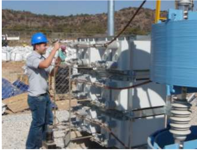
Figure 5.11: Tightening capacitors as per recommended torque levels to bus bar
