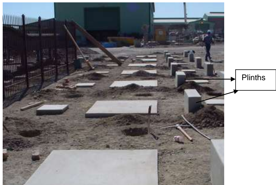
Figure 5.1: Site constructed for reactor and capacitor installation
