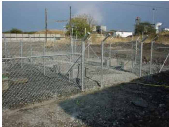
Figure 5.5: Site fencing for harmonic filter installation
