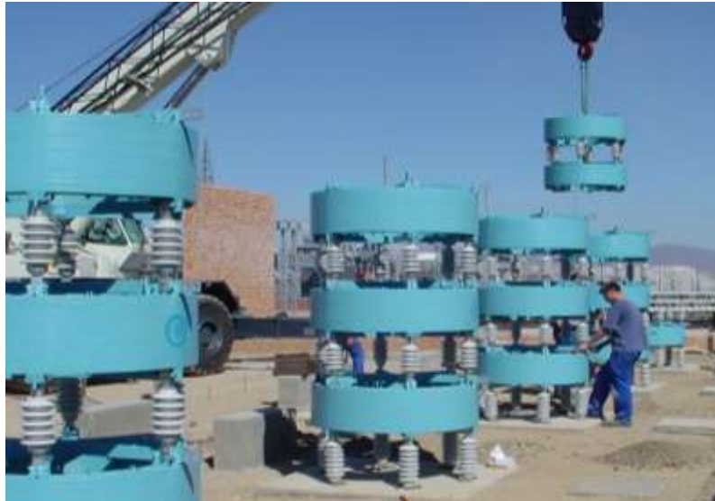
Figure 5.16: Assembled reactors being delivered at site
