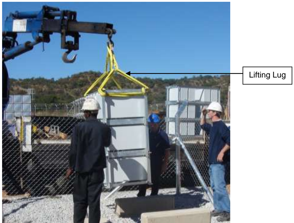
Figure 5.9: Crane downloading capacitor rack to plinth
