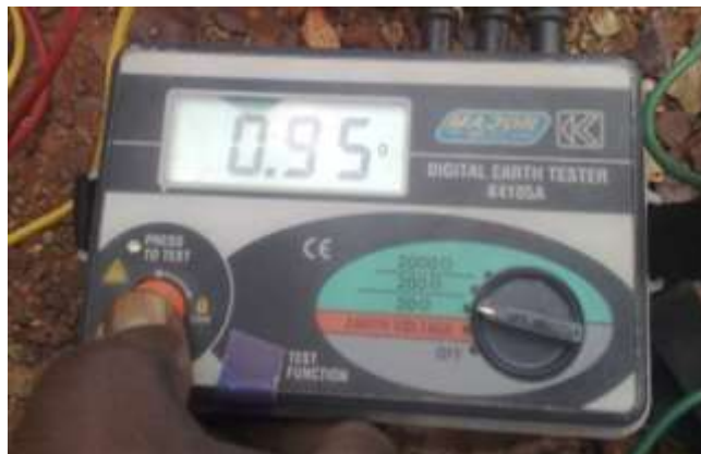
Figure 5.21: Earth continuity test using digital earth tester
