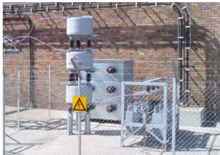
Figure 2.2: Second order harmonic filters at site
