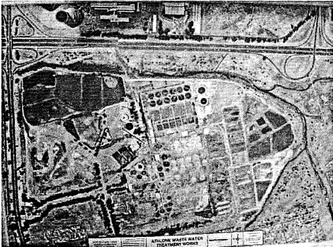
Figure 4. 2: An aerial view of the Athlone Wastewater Treatment Plant.
