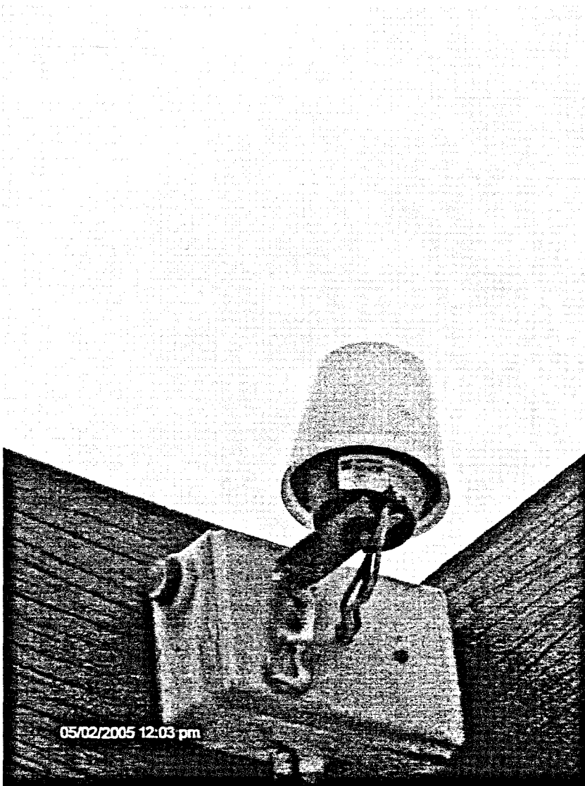
Figure 3.5.8: A light sensor for the outdoor lamps
