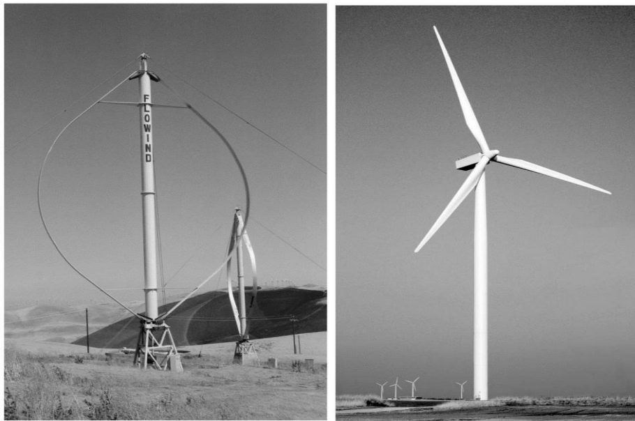
Figure 2.11 Horizontal Axis Wind Turbine (HAWT) and Vertical Axis Wind Turbine (Erich, 2006)
