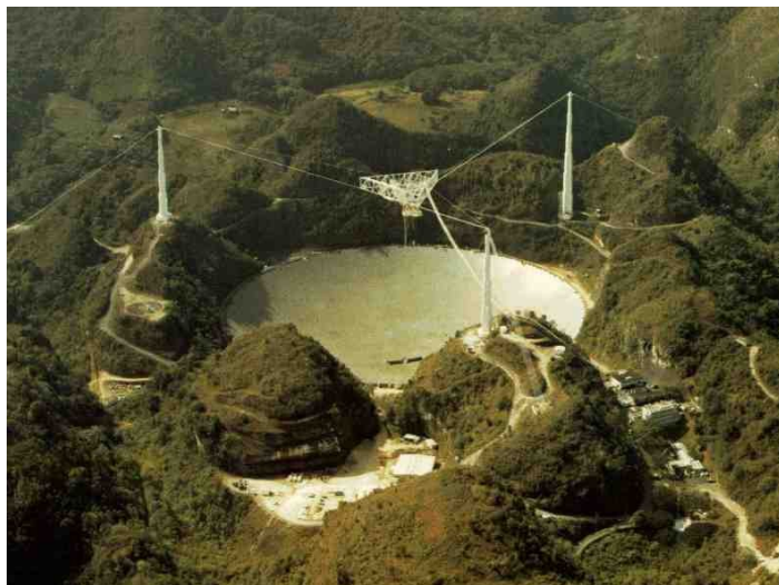
Figure 3.2: Largest single dish radio telescope The 306m in diameter found in Arecibo (Gary, 2005).
