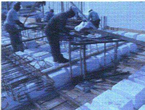
**Figure H.3** Reinforcement and installation of cabling.
