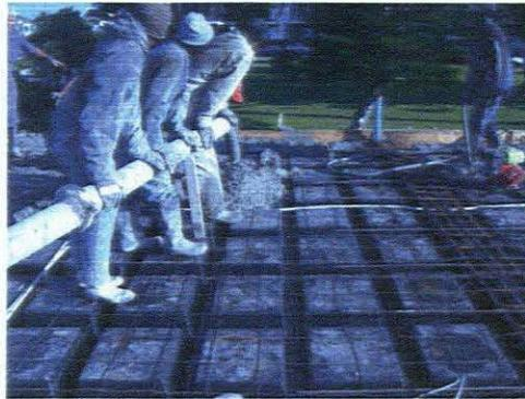
**Figure H.4** Pouring of cement.
