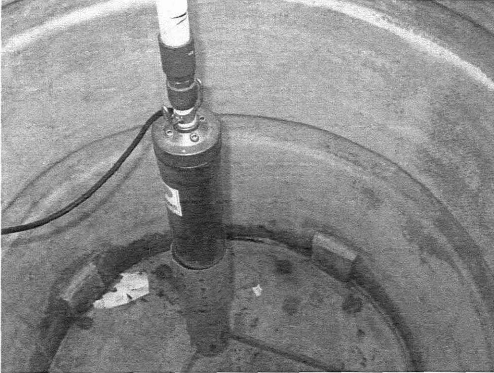
Figure 3.4: Installation of motor/pump unit
