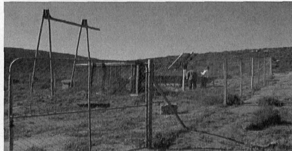
G4: Lepelfontein PV system plant
