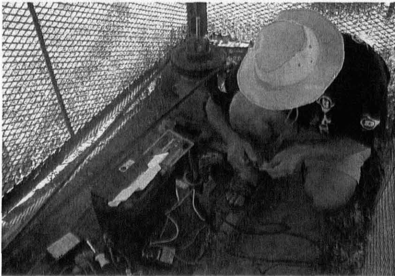
G7: Installation of data acquisition devices
