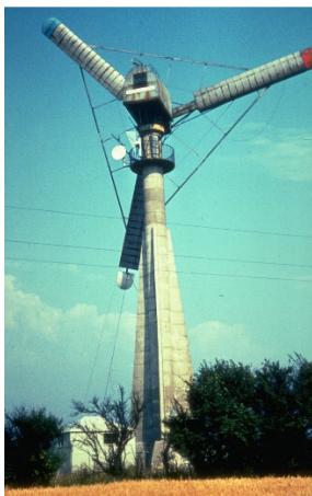
Figure 6: Gedser wind turbine (Denmark)
