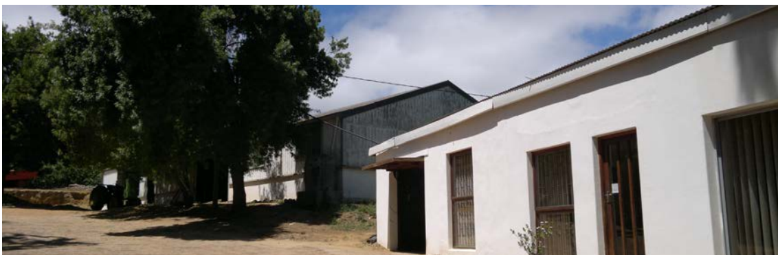
Photo 2.7: On the left behind the tree is the workshop/storeroom and on the right are the offices.
