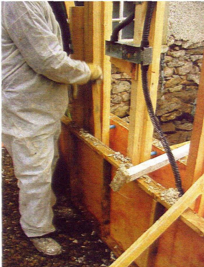
Figure 5.3.4.1: Compressing a hemp mixture into a wall mould (Allin 2005:130)
