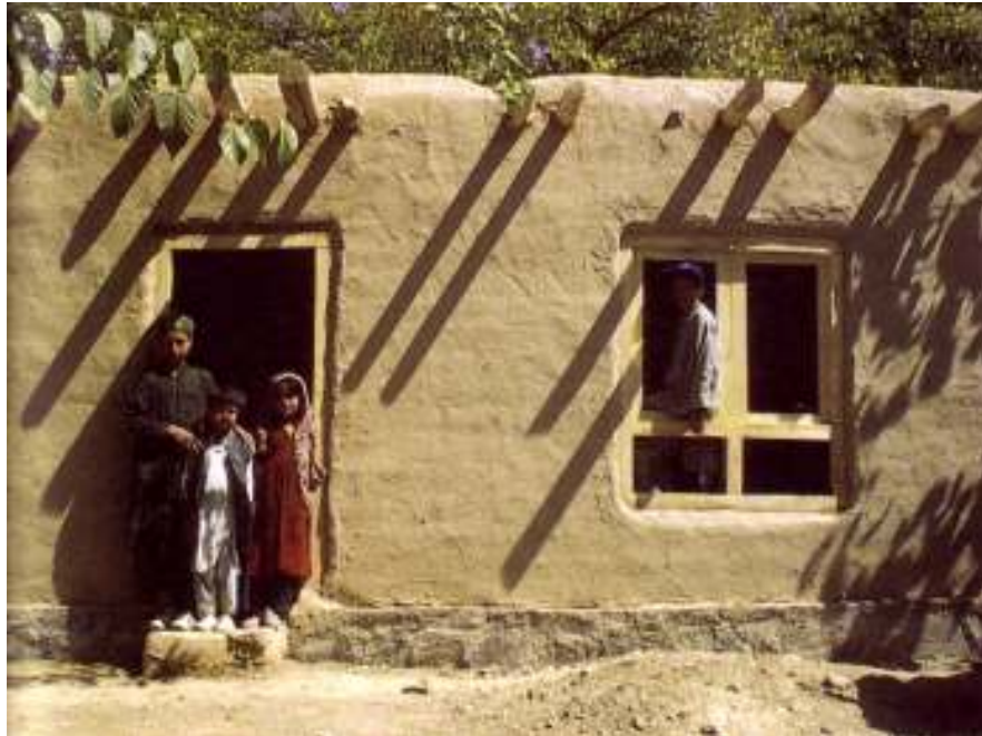
3.16 Adobe Shelter by Shelter For Life, 2002 (Architecture for Humanity, 2006: 133)
