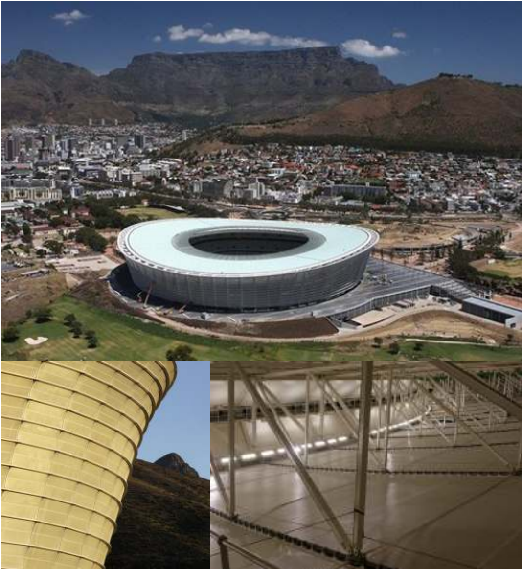
Fig 3.46 The Greenpoint Stadium, Cape Town (Source: www.inhabitat.com )
