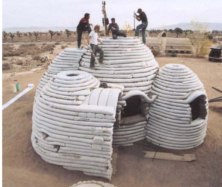
Fig 3.18 Cal-Earth Ecodome construction (Source: www.vestaldesign.com )
