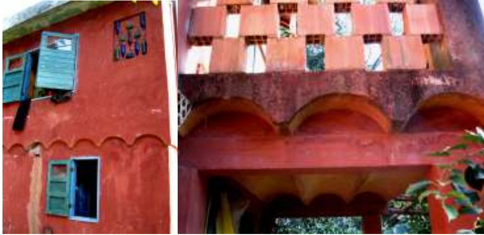
Fig 3.23 Textile-reinforced vaulted concrete shell panels at TIBA, Brazil (Photos: F.De Flamingh)
