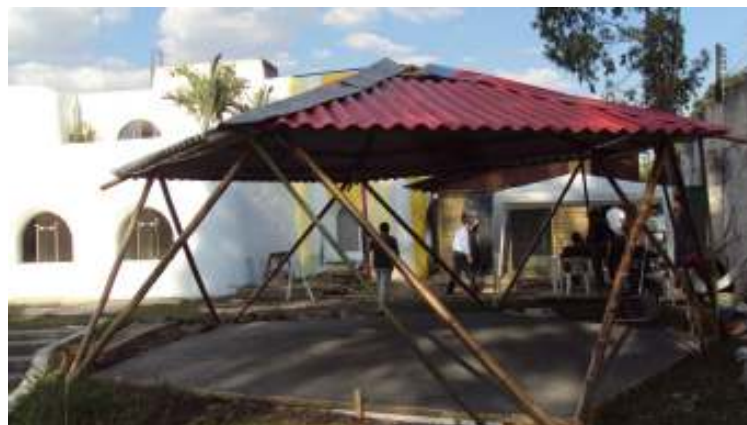
Fig 6.3 Bossa Nova Shelter bamboo frame and roof (Source: www.sersustentavel.com.br )
