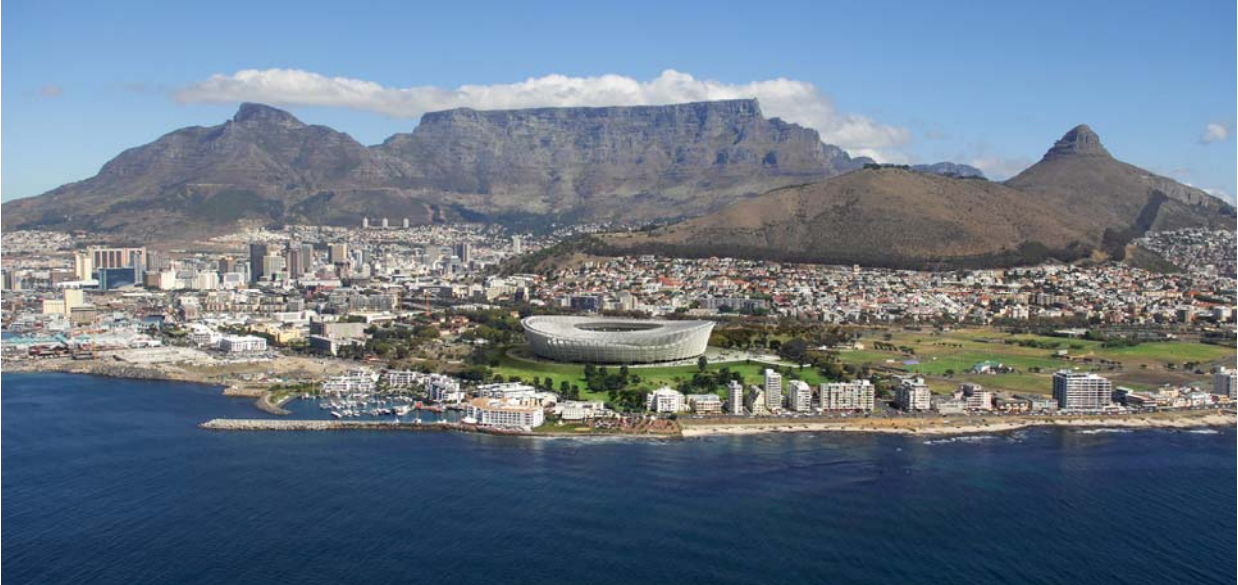
Figure 2.11 Panoramic view of the completed Greenpoint Stadium (source: City of Cape Town)
