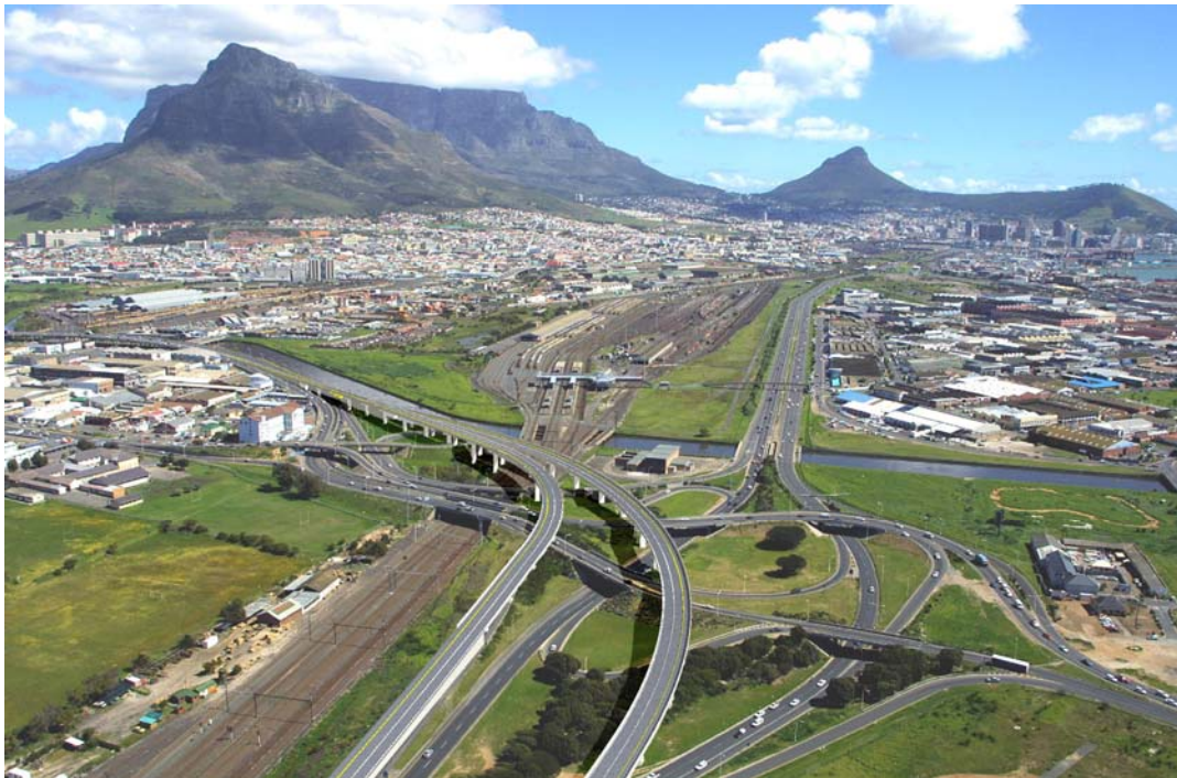
Figure 2.10b Ongoing upgrading of road infrastructure – after completion (source: Donald Cupido – City of Cape Town)
