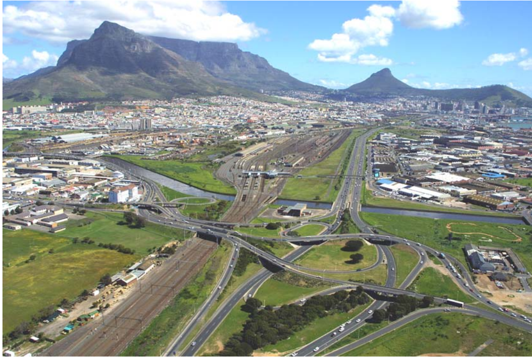
Figure 2.10a Ongoing upgrading of road infrastructure – before construction (source: Donald Cupido – City of Cape Town)
