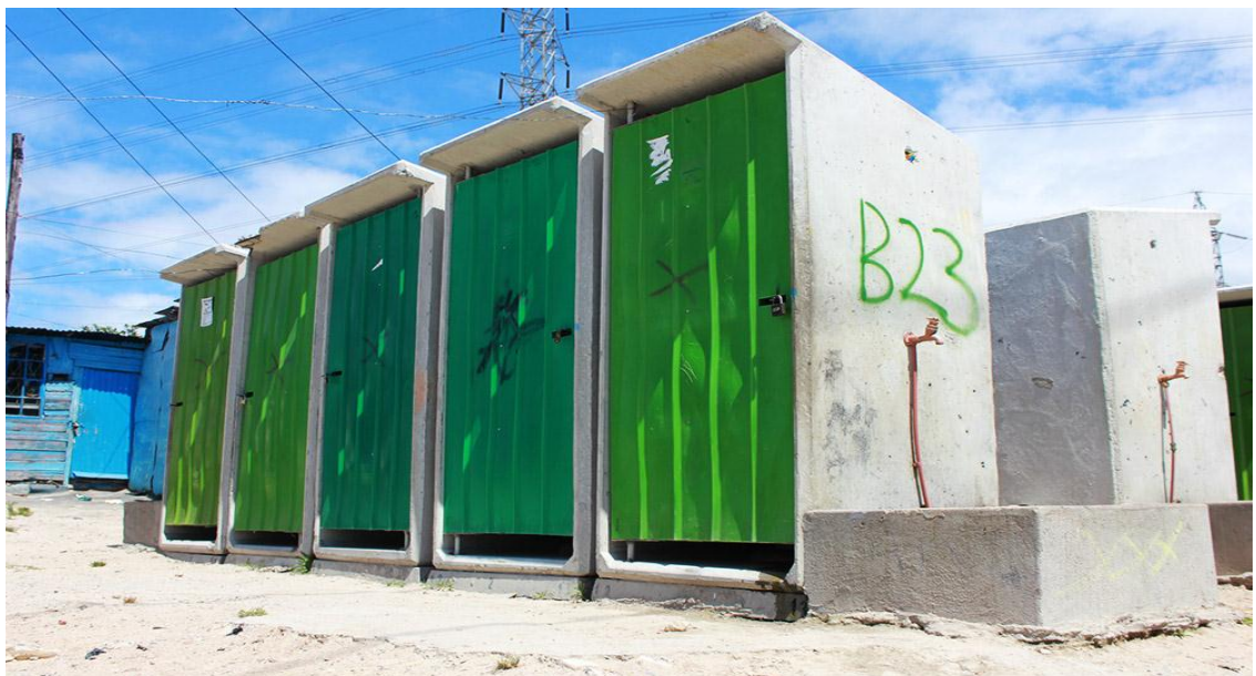
Figure 6: Public toilets in Khayelitsha
