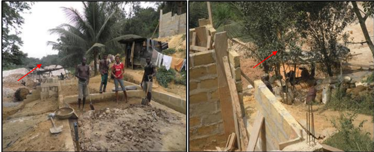
Erections of buildings close to small-scale mining (indicated in red arrow) at Nkamponaase. Lack of accessibility and affordability can result in the use of unsuitable spaces as a way of coping
