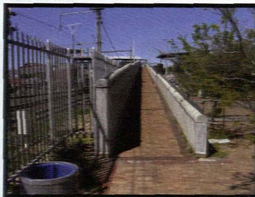
Figure 4.23: Ramp at Mowbray Public Transport Interchange
