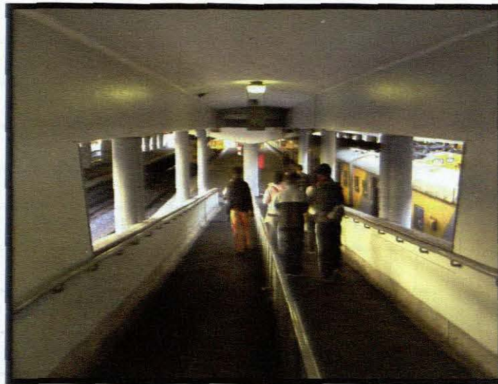
Figure 7.4: Ramps at Cape Town train station do not have sufficient landings.
