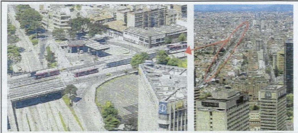
Figure 5.2: TransMilenio bus system components (Targa, 2003: 24).
