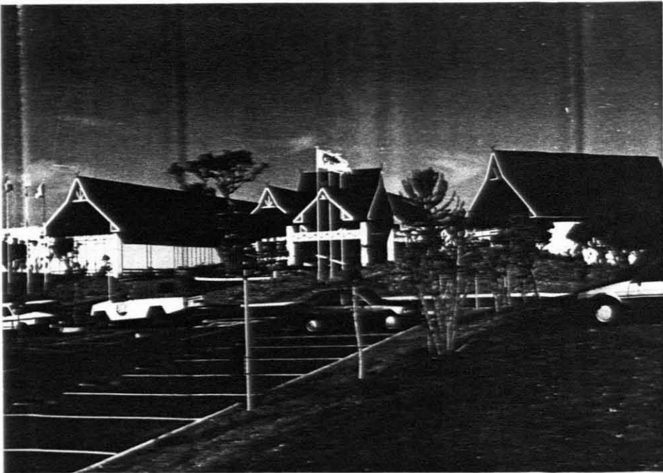
FISH RIVER SUN HOTEL COMPLEX
