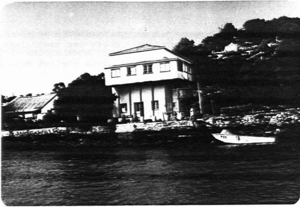
PORT CAPTAIN'S OFFICE AND MILL
