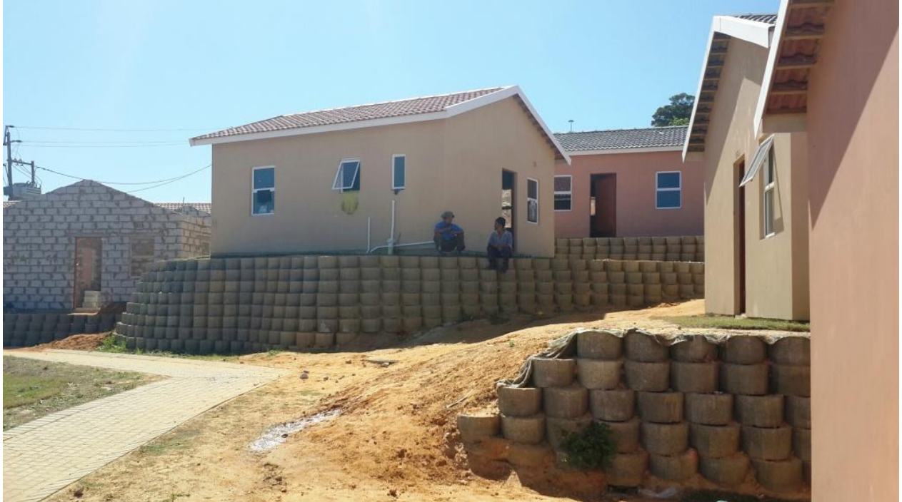
Figure 3.16: Oupad Knysna PHP Housing Project
