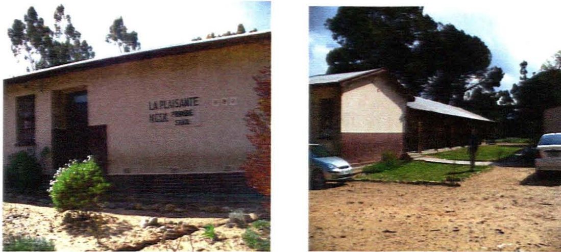
Figure 5.1: La Plaisante Primary School.
