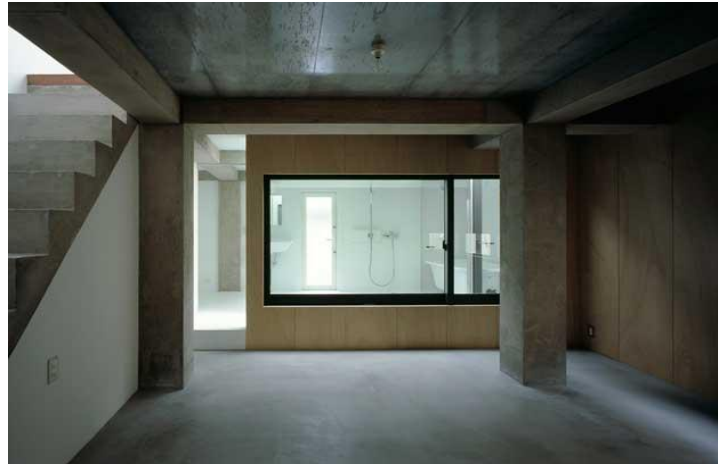
Figure 1.3: Newly constructed concrete column constructed on site
