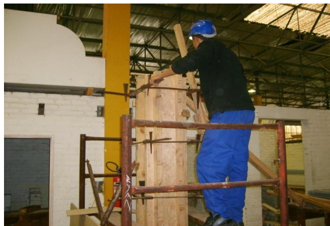
Figure 1.2: A student constructing a simulated concrete column in the workshop
