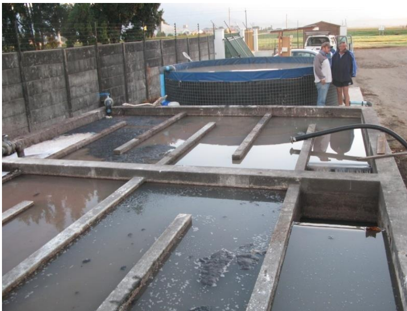
Figure 3.3. The sedimentation dam in front and the stock dam at the back
