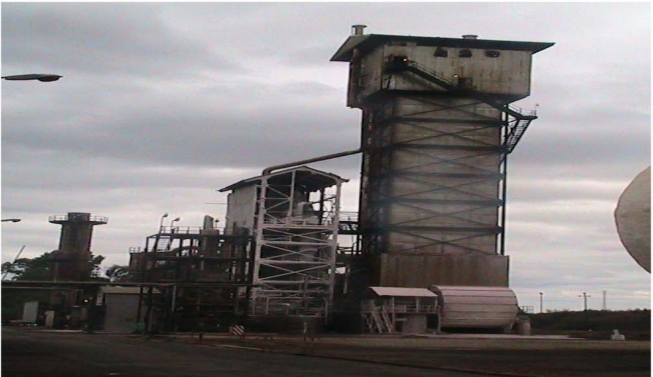
Figure 19: Ammonium nitrate plant at S.C.I Date taken: 24 Sept 2012
