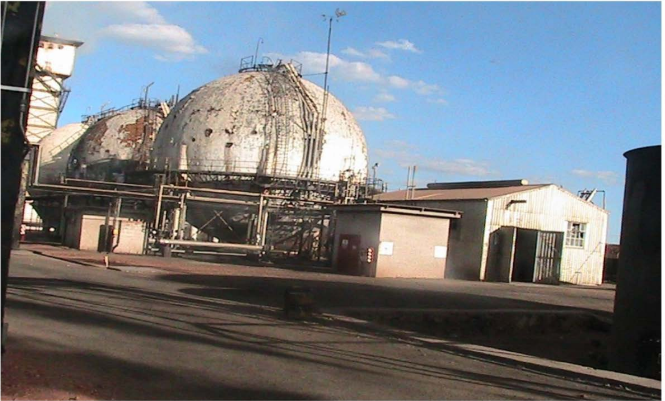
Figure 17: Ammonia storage tanks at S.C.I Date taken: 24 Sept 2012
