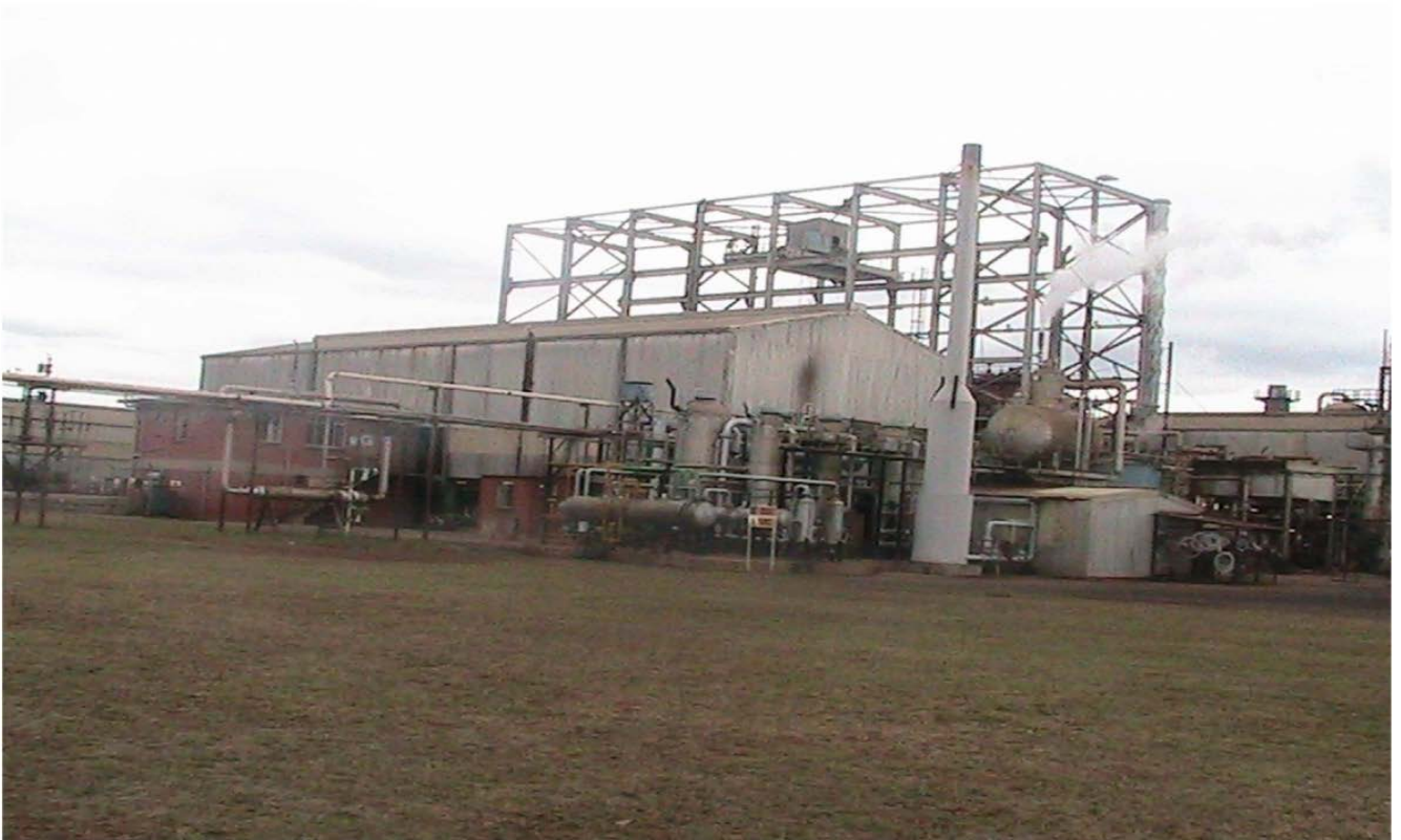
Figure 16: Ammonia plant (Loop) at S.C.I Date taken: 24 Sept 2012
