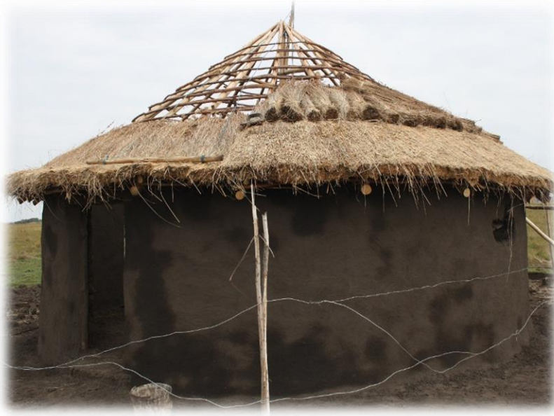
Figure 8.10: Rondavel-type accommodation being built in Ndengane
