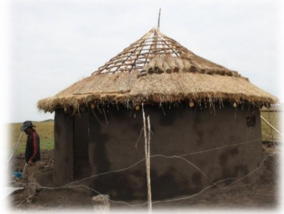
Figure 6.6 (d) Homestay at construction stage
