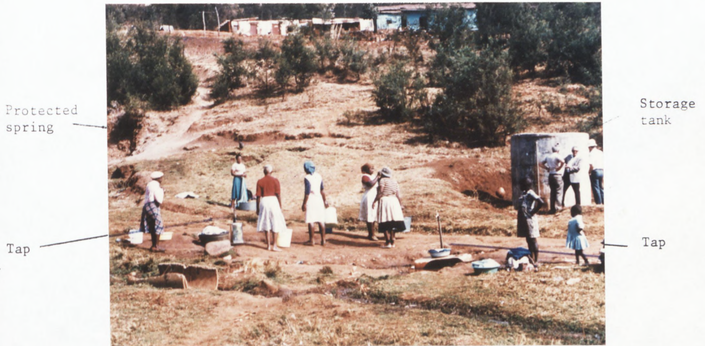
17. Kwashishi - Protected spring with storage tank and two taps.
