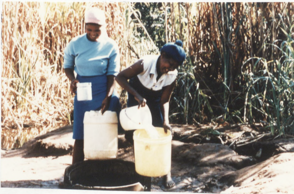
12. Driefontein - Concrete pipe sunk in bed of small stream. Water is clear, but has more than 500 faecal coliforms/100 ml . This is the water source for the village.
