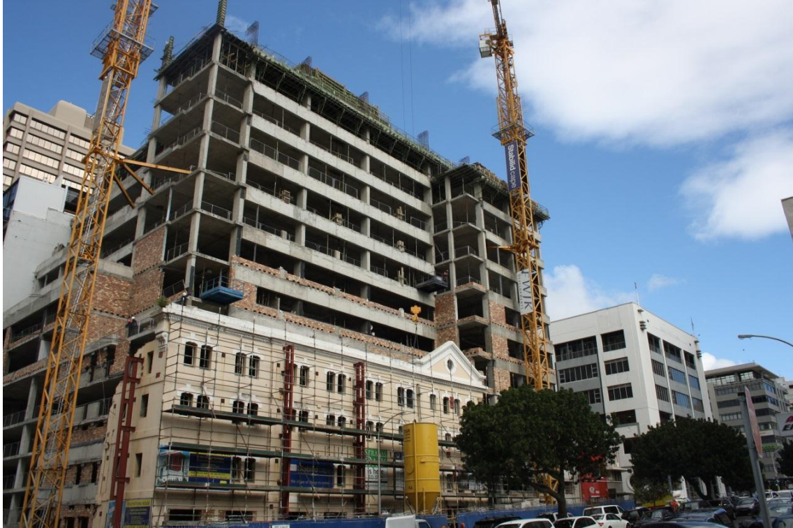
Plate 5.9: Incorporating the existing building facade - heritage requirement (Touchstone Office Development, Cape Town Urban Centre, April 2015)
