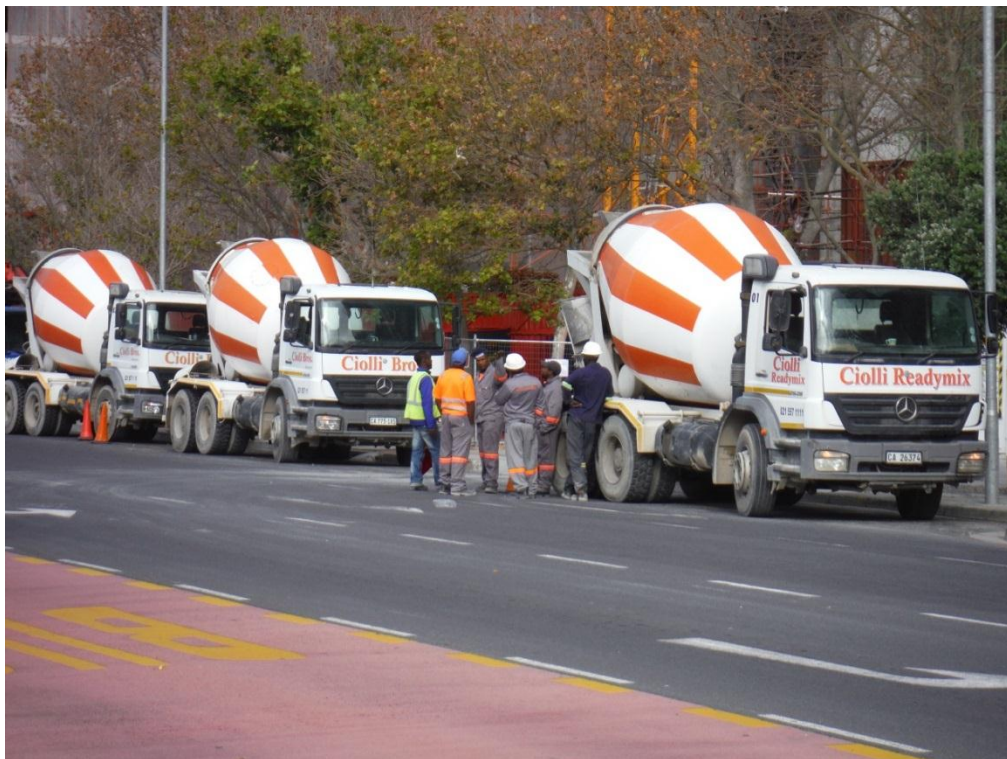
Plate 5.14: Ready-mix concrete delivery (The Towers, Cape Town Urban Centre, March 2013)
