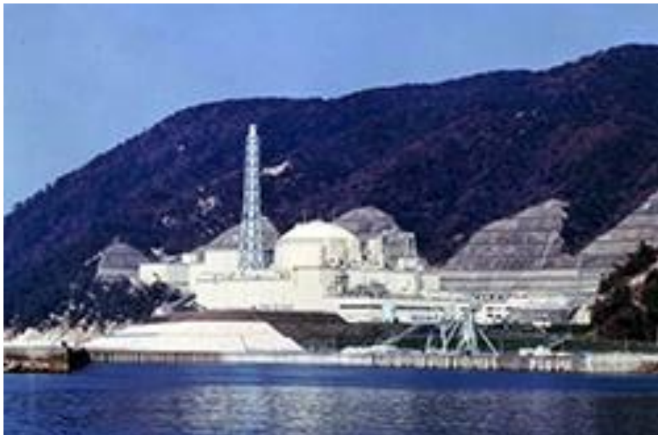
Figure 2.12: The Japanese Monju loop type sodium-cooled fast reactor (IAEA, 2013)
