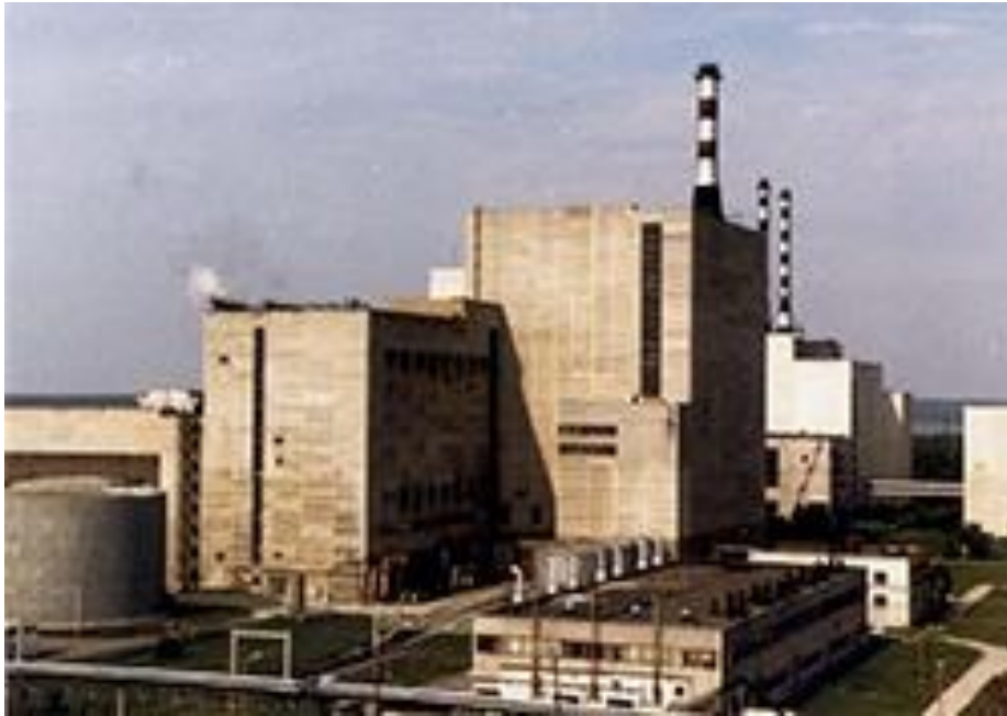
Figure 2.11: The Russian Sodium-cooled fast reactor BN-600 in operation since 1980 (IAEA, 2013)
