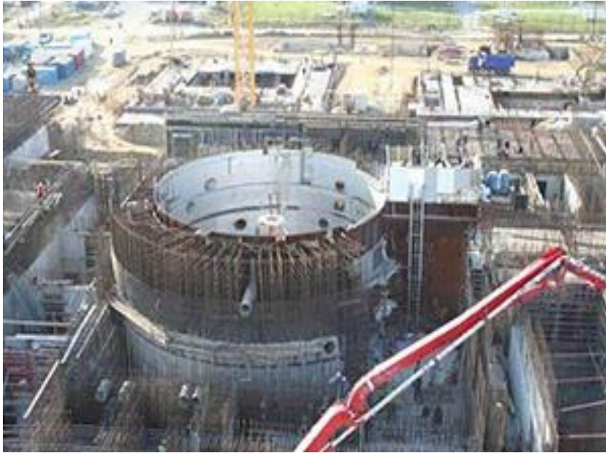
Figure 2.14: The Russian sodium-cooled fast reactor BN-800: construction initiated in July
