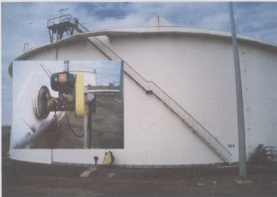
Figure 6.2. Petroleum storage tank. Inset: Mixer motor
