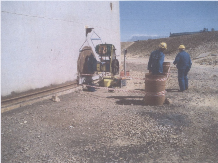
Figure 3.5 Motor and mechanical coupling of the stirrer
