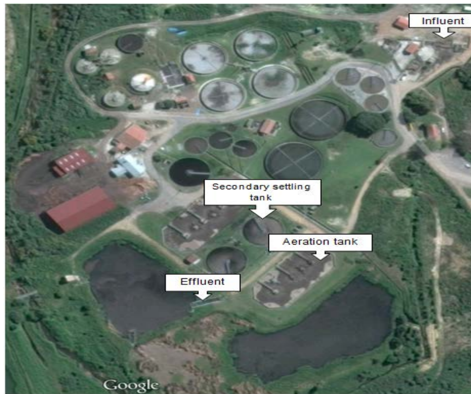
Figure 2.1: Stellenbosch wastewater treatment plant (WWTP) sampling sites, Stellenbosch (GPS: -33.9447525, 18.8231056) (Google Maps, 2015).
