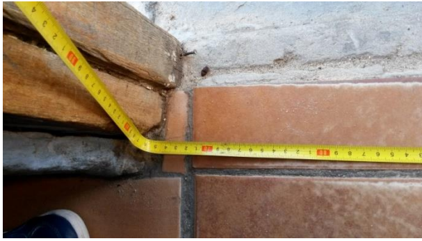
Onsite Image 33: Clear opening width of the entrance door.
