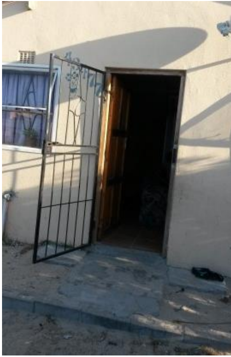
Onsite Image 30: Entrance door to the house where the residents have built an extended stepped access to allow small children easier access to the house.
