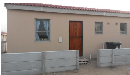
Onsite Image 14: Various solutions have been put in place at the houses to overcome the sandy entrance and the high step at the entrance.
