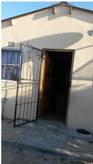
Onsite Image 4: Entrance door to the house where the residents have built an extended stepped access to allow small children easier access to the house.
