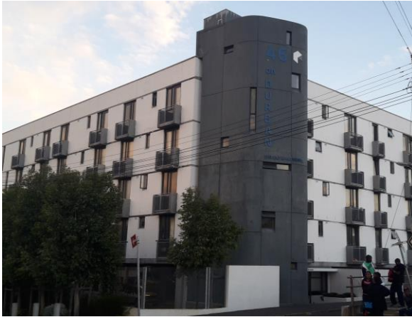
Figure 3.16: Student Residents in Mowbray, Cape Town, which has been constructed with modular, precast 'building blocks'. (Fransolet, 2014)
