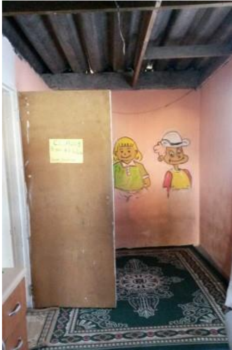
Onsite Image 52: One of the classrooms that was an original bedroom.
