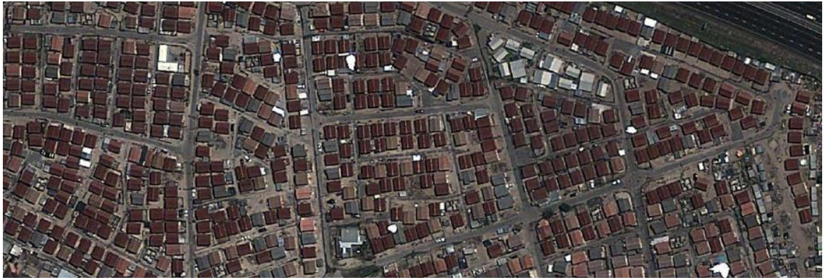
Figure 1.2: Aerial view of New Rest settlement just off the N2 highway, approximately 20km from the city centre of Cape Town. New Rest is an example of the mass construction of low-cost housing, where little attention appears to have been paid to the design of the area and the importance of creating communities. Image from: Google Earth, New Rest Settlement, Cape Town, South Africa.
