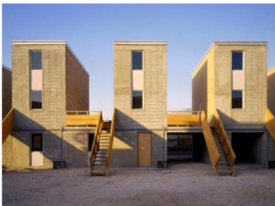
Figure 3.6: Final construction of the social housing in Chile, by Elemental, where the climate is desert like. (ArchDaily, 2008)
