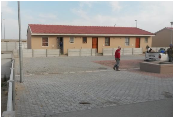
Onsite Image 56: Central parking area with drainage in the centre of the lot and directly along the walkway leading to this area.
