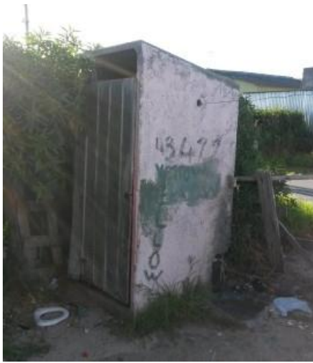
Onsite Image 45: Toilet facilities are in the form of an outhouse.
