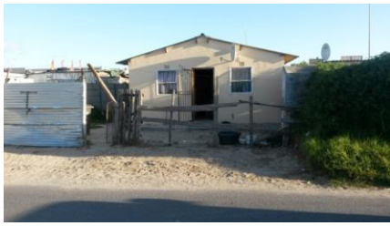
Onsite Image 3: Street access to the house.
