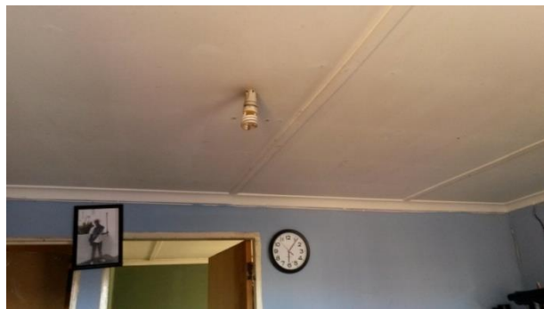
Onsite Image 43: Ceiling installation that was done by the residents.
