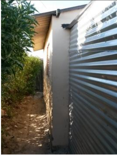
Onsite Image 47: Image of where the backyard dwellers have built up against the back of the house to secure their shacks.
