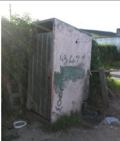
Onsite Image 5: Toilet facilities are in the form of an outhouse.
