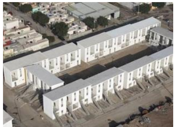
Figure 3.7: Final construction of low-cost housing in Mexico by Elemental. Photos by Ramiro Ramirez (Bustler, 2010)
