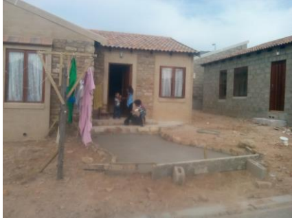
Onsite Image 26: Example of what residents have put in place to overcome the lack of pedestrian access to their houses. Residents also erected washing lines, in the absence of sufficient servicing facilities in the area to meet their needs.
