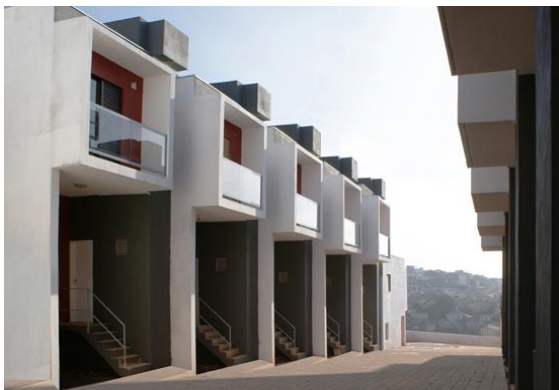
Figure 3.4: Image of Box Houses in São Paulo, Brazil by Yuri Vital. (Damen, 2009)
