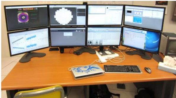
Figure 2.6, Blanco Control Room Osuwomeninphysics, 2013
