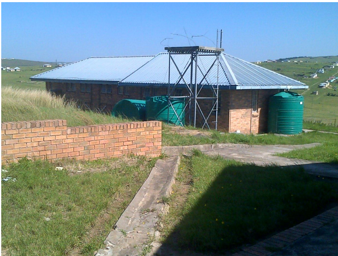
Figure 7: Example of the water supply for the clinic.
