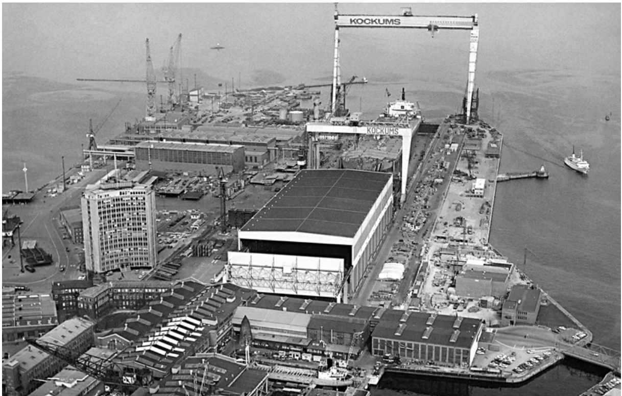
Figure 3.1: Kockums shipyard in 1974. (City of Malmö, 2014)
