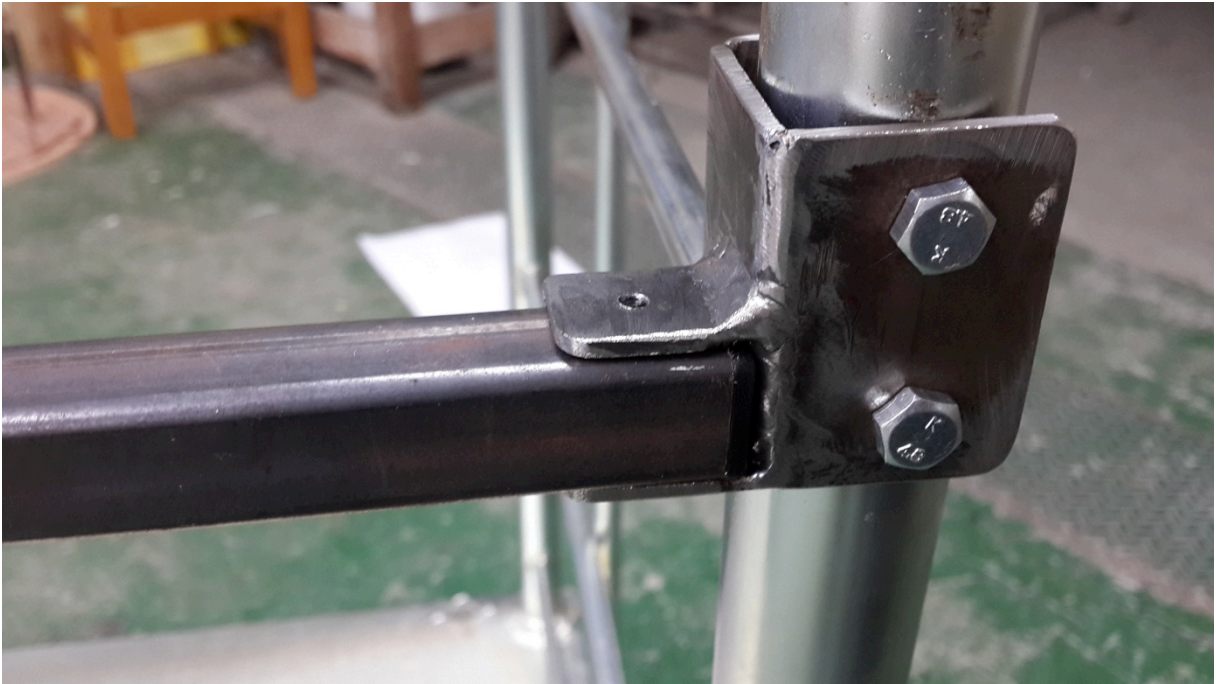
Figure 5.5: Bracket Coupling & Side Panel Pole. (Donnoli, 2014)
