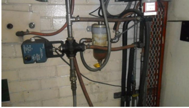
Figure 3.4: 2nd room AVL container filled with fuel feed by the fuel pump
