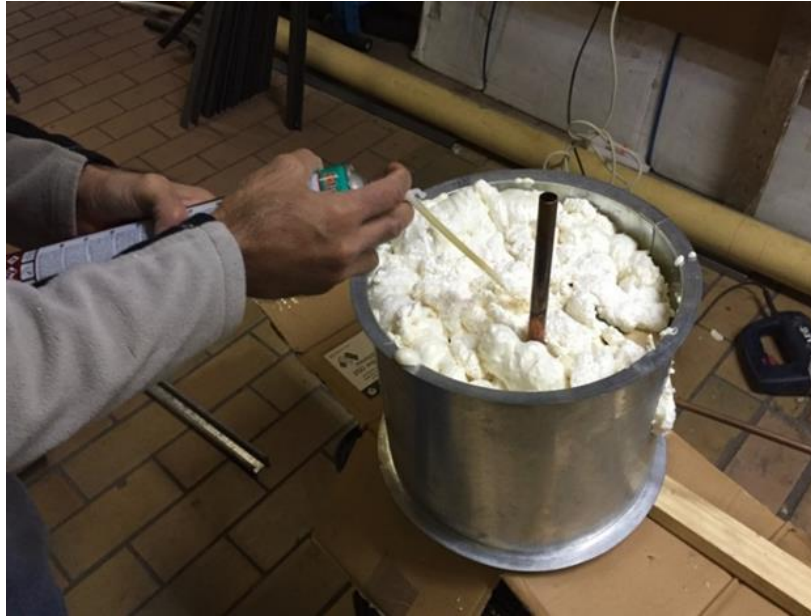
Figure 3.21: The tank being insulated during its construction.
