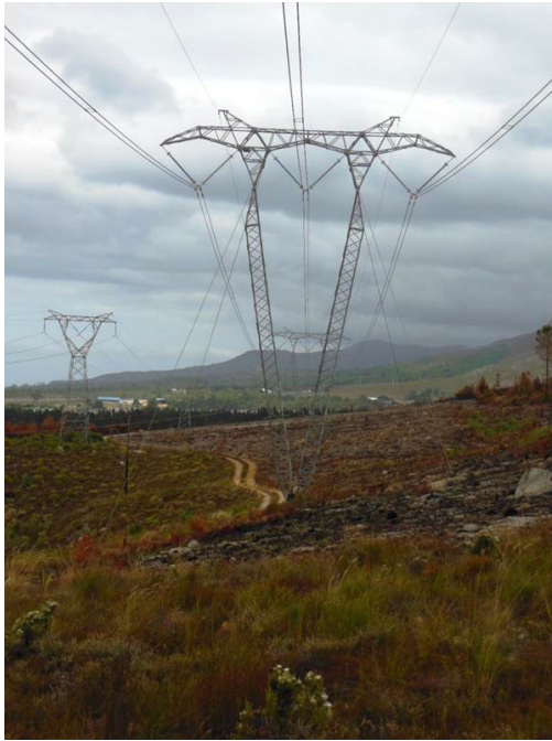
(a) View of the closest 400 kV line pylon.
