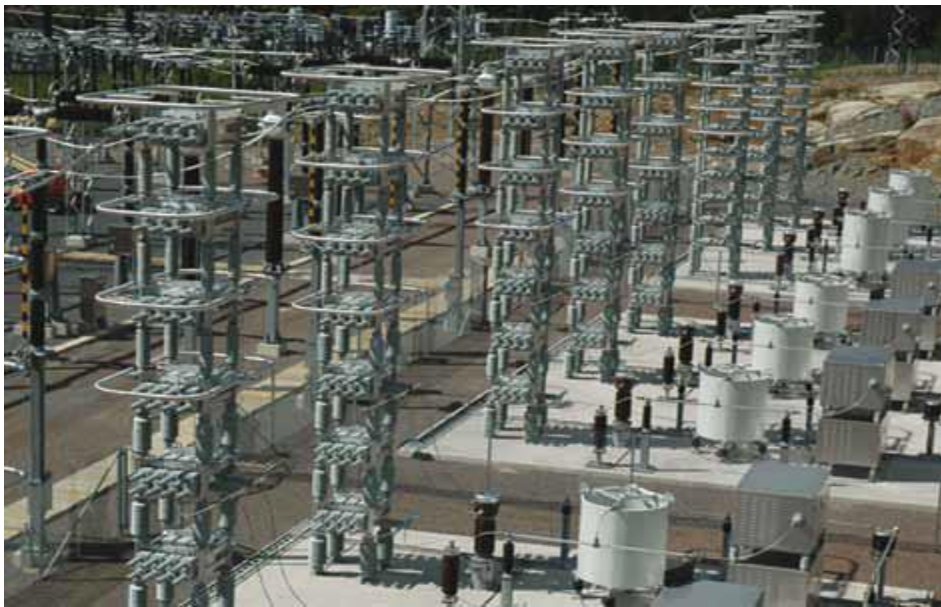
Figure 4. 7: A typical AC harmonic filtering system (ALSTOM, 2010)
