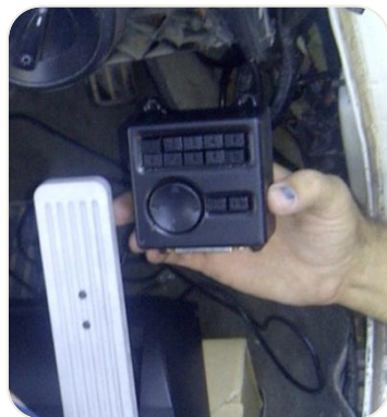
FIGURE 4.27: PLACING THE SWITCH BOX (Author, 2013)
