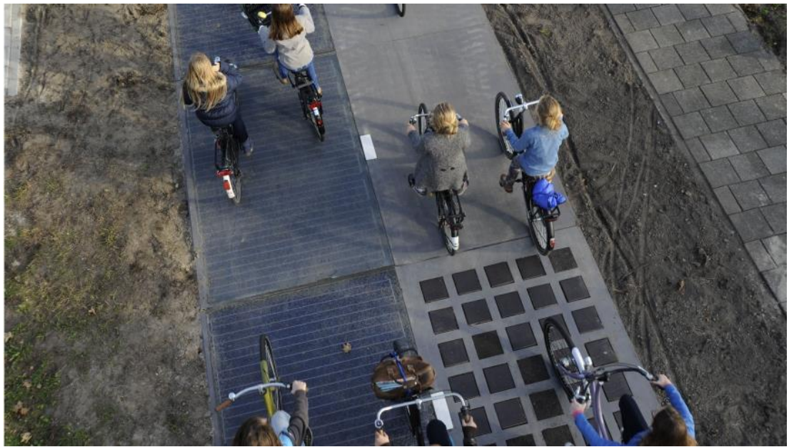
Figure 1.2: Cyclists ride over a stretch of a new cycle path surfaced entirely with solar panels in the Netherlands. (Hruska, 2014a)
