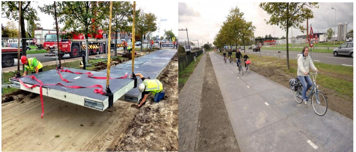
Figure 2.3: The world's first solar-paneled road in the Netherlands
