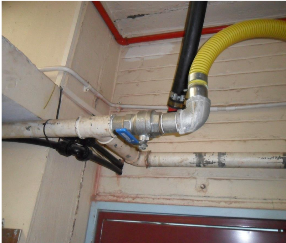
Figure C5: Connection to the municipal mains
