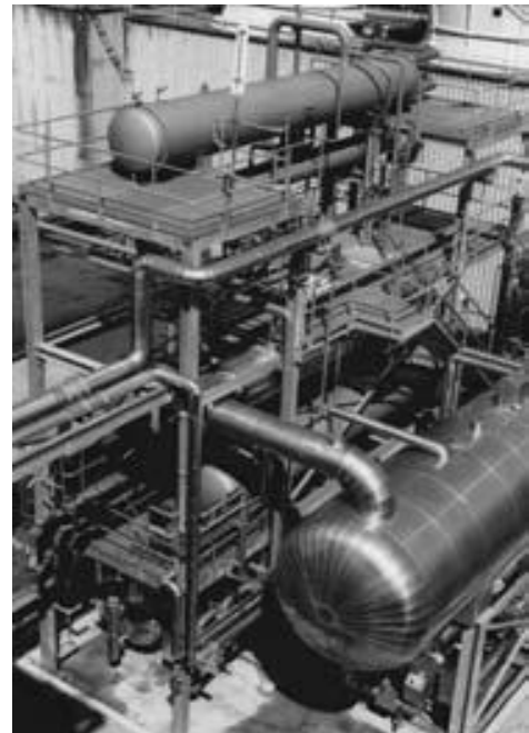
Figure 2.4: A VARS of 2700 kW at -30\text{ }^{\circ}\text{C} installed in a refinery in Germany (Dinçer & Kanağlu, 2011,183-b)
