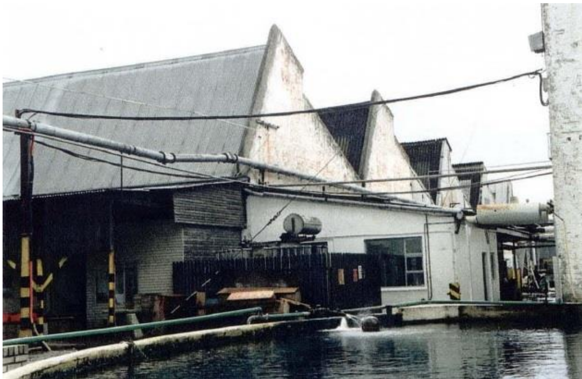
The Sawtooth building before adaptive reuse (source: Hart & Halkett, 1998)
