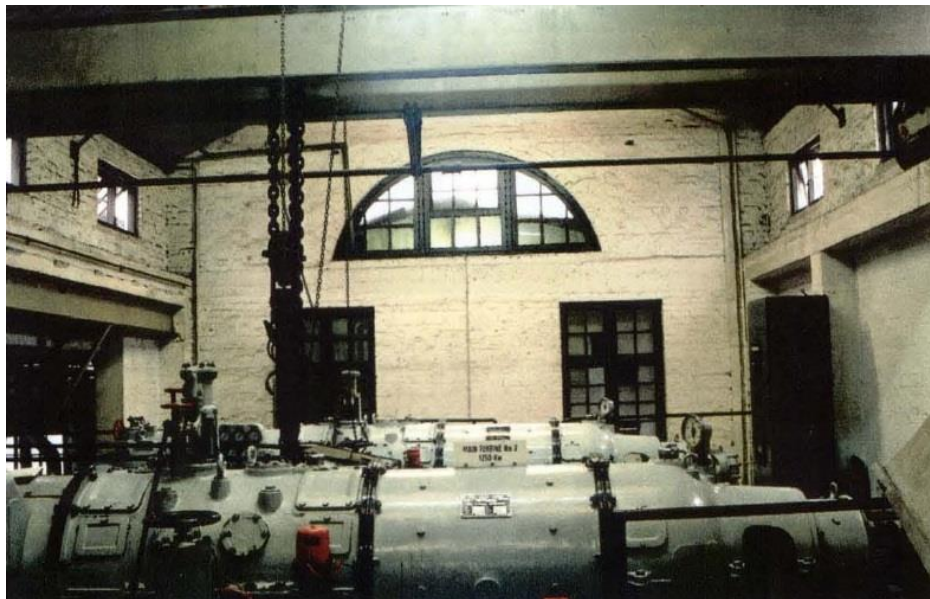
Figure 4-34: Main turbine hall showing the turbines constructed by De Laval and Ljungstrom (source: Hart & Halkett, 1998)
