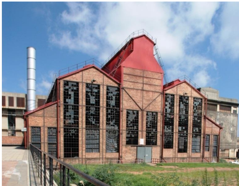
Figure 2-26: The front façade of the Turbine Hall before redevelopment (source: Schoemaker, no date)
