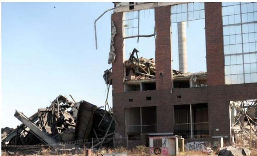
Figure 2-28: The ruins of the Orlando power station (source: The Citizen, 2014)
