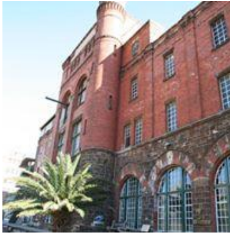
Figure 2-11: Castle Brewery building, Cape Town
