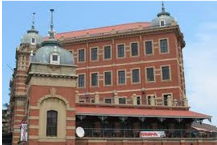
Figure 2-4: Preserved façade of the old Durban Station
