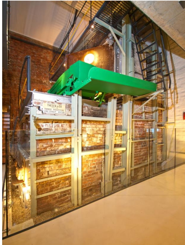
Figure 4-31: The boiler after reuse (source: Flemming, no date)
