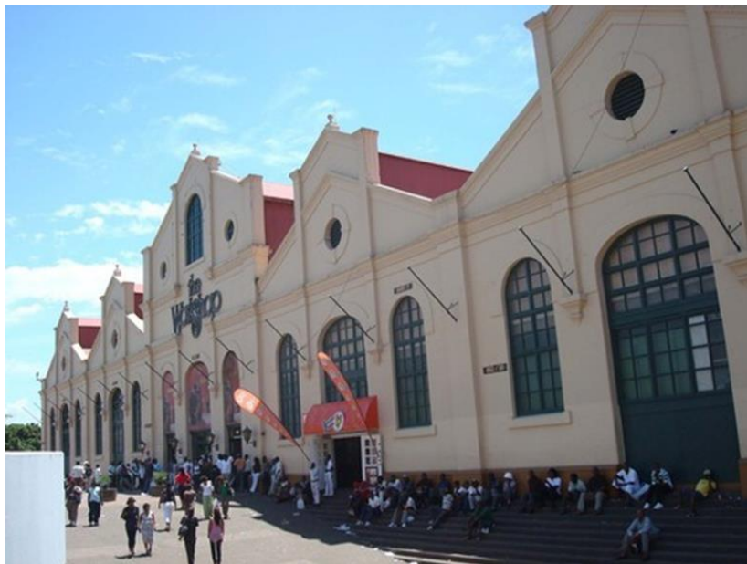
Figure 2-5: Durban railway sheds adapted for reuse as a shopping centre (source: The Workshop, no date)
