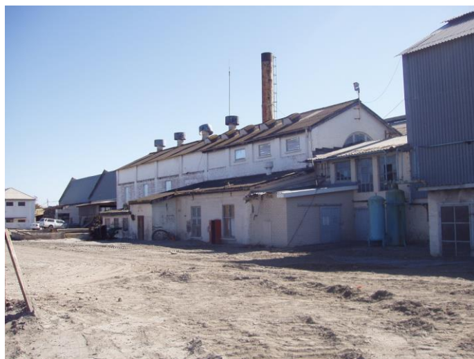
Figure 4-4: Southern elevation of the Thesen Island Power Station before reuse (source: Louw, no date)
