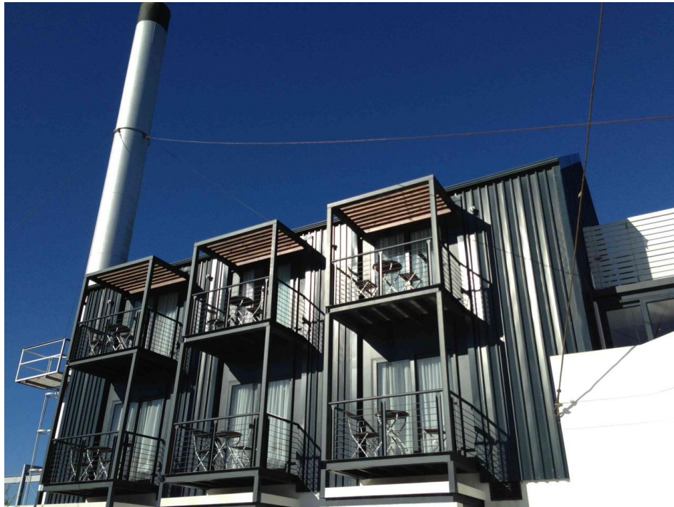
Figure 4-24 Brise soleil or shading devices used on the northern façade which houses the guest bedrooms (source: researchers own 2013)
