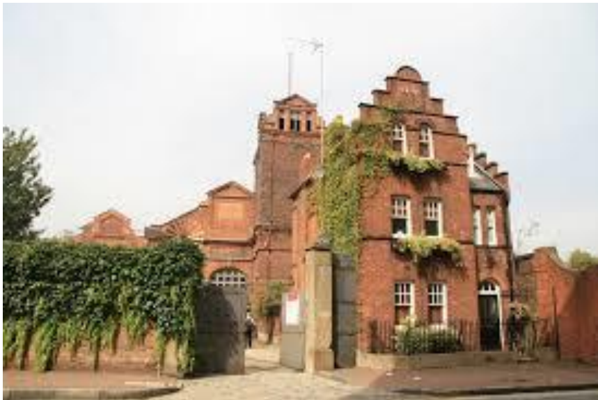
Figure 2-22: Wapping Power Station, UK (source: Monk, no date)
