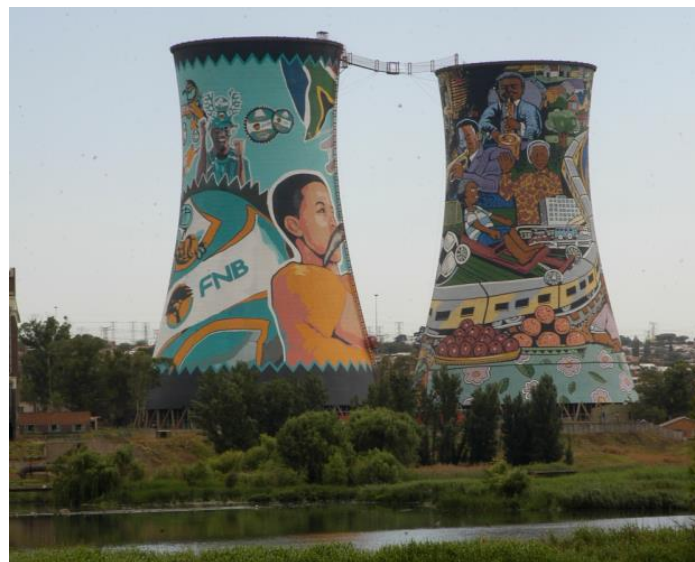
Figure 2-29: Orlando cooling towers (source: Gauteng.net)
