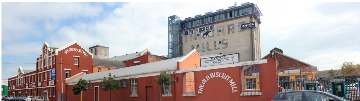
Figure 2-12: Old Biscuit Mill in Cape Town
