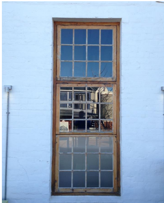
Figure 4-28: An original timber window casing retained for reuse (researcher's own, 2012)
