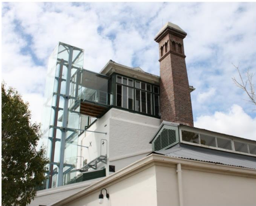
Figure 2-13: Fagan's 1993 glazed insertions at the Newlands Brewery in Cape Town and the reconstructed chimney (source: Barker, 2009)
