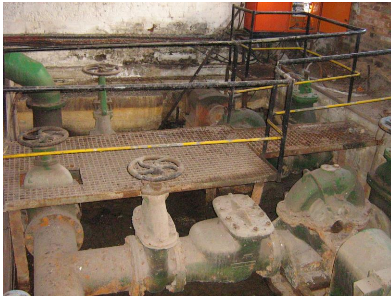
Figure 4-29: The area to become the hotel lobby before reuse (source: Louw, no date)
