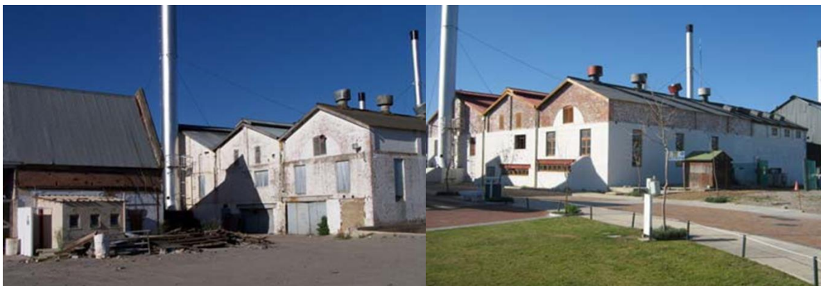
Figure 5-1: Before and after initial preservatory work to the power station
