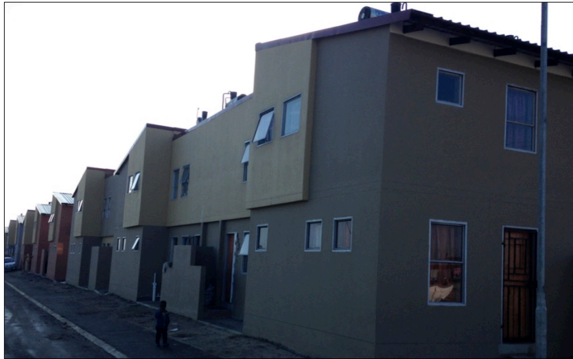
FIG 4.1 N2 Gateway Phase 3 housing. (Author, 2015)
