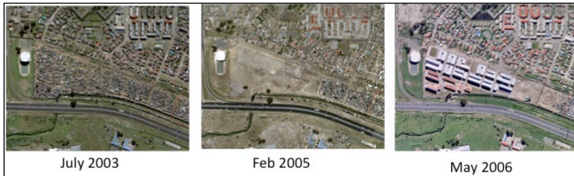
FIG 5.7 Progress of Phase 1 of the N2 Gateway project (City Maps, 2015)
