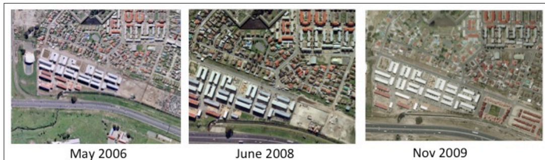
FIG 5.8 Progress of Phase 2 (2006-2009), adjacent to the completed phase 1 (City Maps, 2015)
