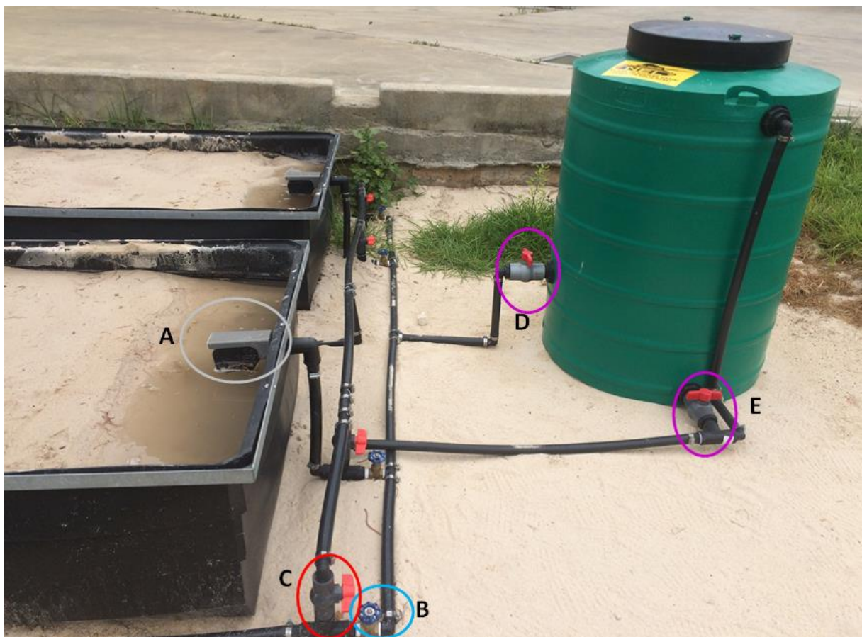
Figure 3.4 A picture depicting the inlet manifold and float valves for the BSF filter modules plus the 500 L holding tank
